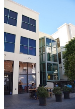
Access from alleyways and courtyards
