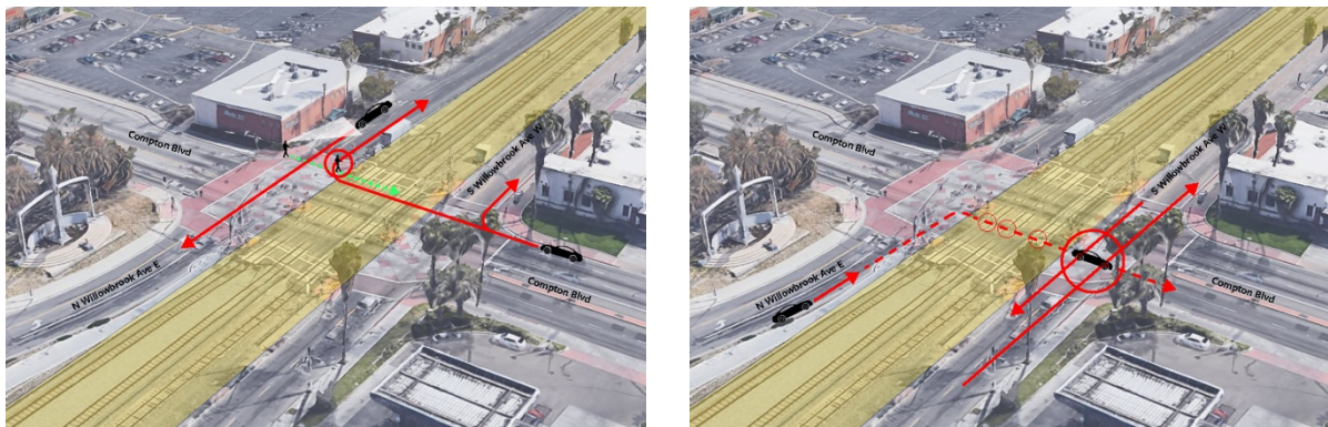
Figure 5-8. Common Safety Issues at Willowbrook Avenue intersections.
