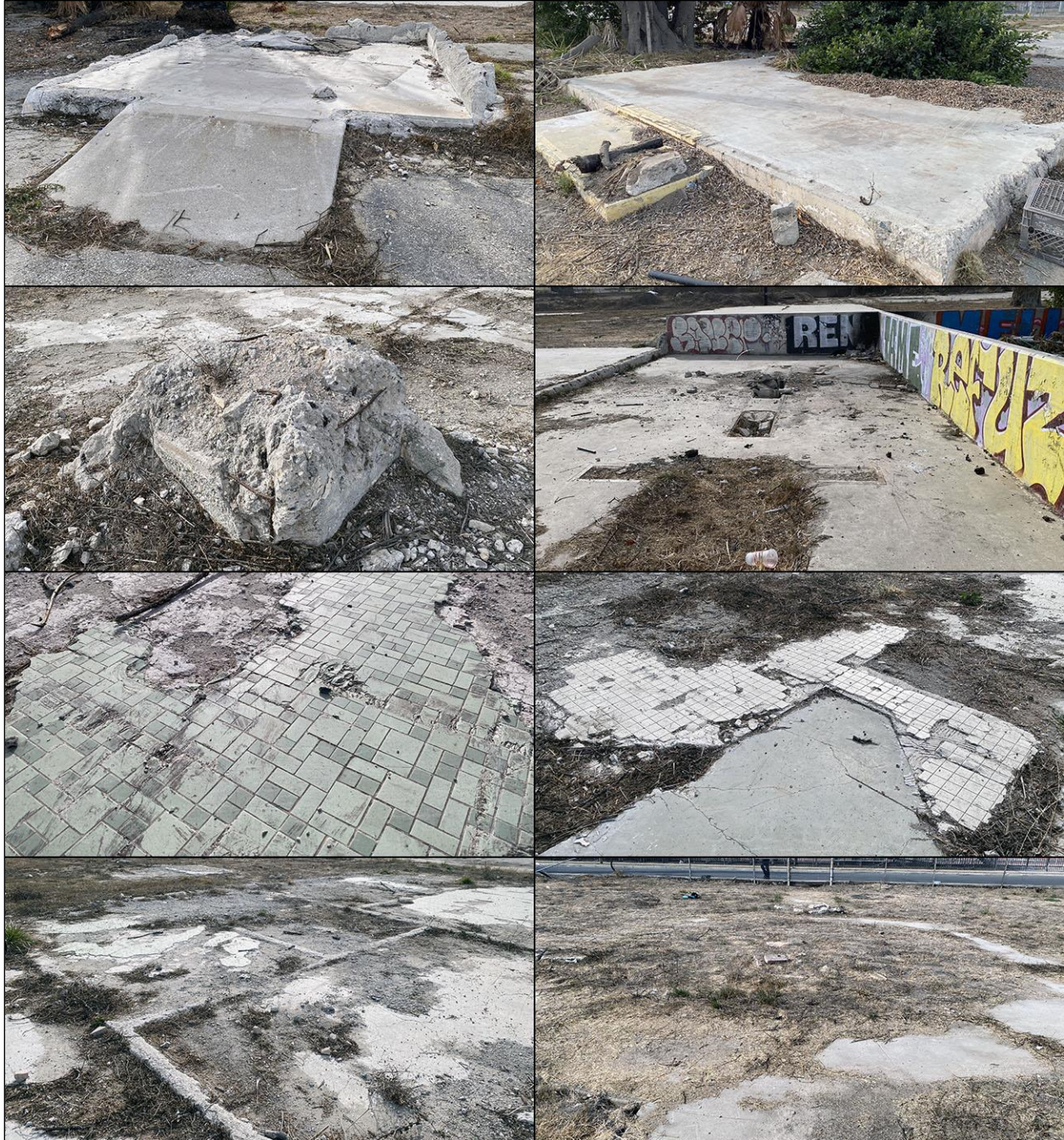
Structural remains at the site. Clockwise from top left : CF-07, view to south; CF-06, view to southwest; bays in CF-04, view to south; CF-04 white tile, view to southwest; courtyard circle, view to west; room divisions in CF-01, view to southeast; CF-01 green tile, view to south; CF-04 column remains, view to southwest.
