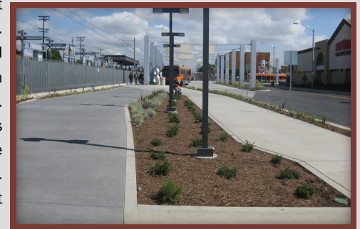
MLK Jr. Transit Center Pedestrian Walkway
