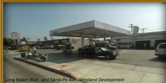
Long Beach Blvd. and Santa Fe Ave., Westland Development
